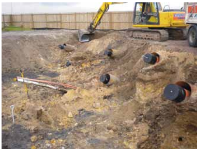
Figure 10. Completed HDD lines.
