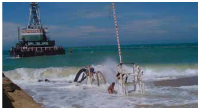
Figure 7. Roncador surf trenching.
