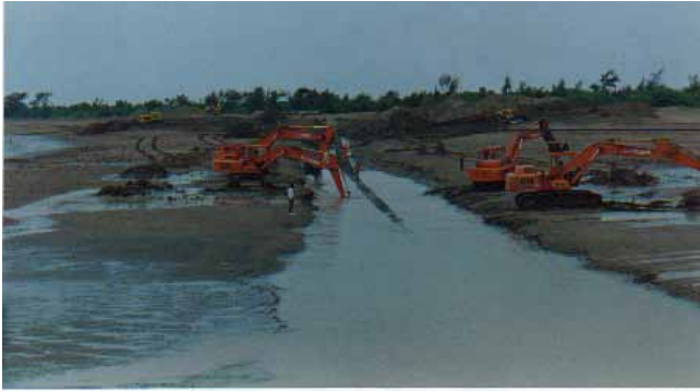
Figure 2. SBHT line excavators assist.
