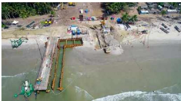
Figure 2. The layout on the beach for the onshore operation, including the failed shallow water spread to the left.
