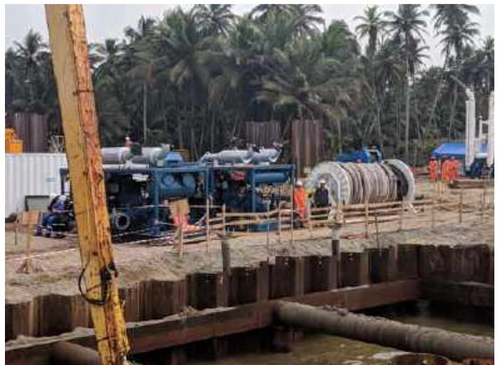
Figure 3. Pumps at the edge of the suction pit.
