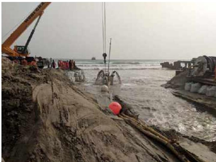
Figure 1. Completed pre-trenching, and the start of post-trenching.
