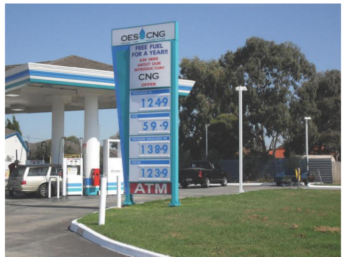
OES CNG SmartGas Refuelling Station
